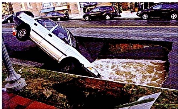
A car falls into a sinkhole
