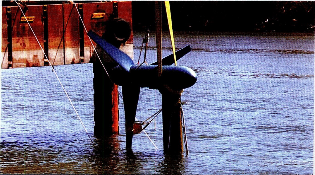
Workers lower a tidal power turbine into the East River.
